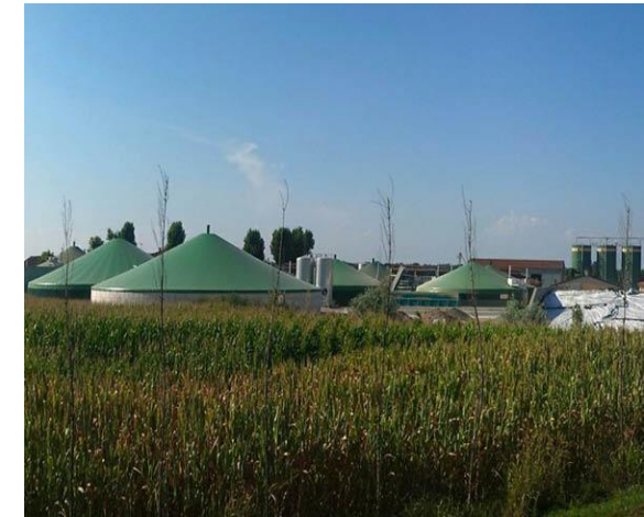
Anaerobic Digestion facility
